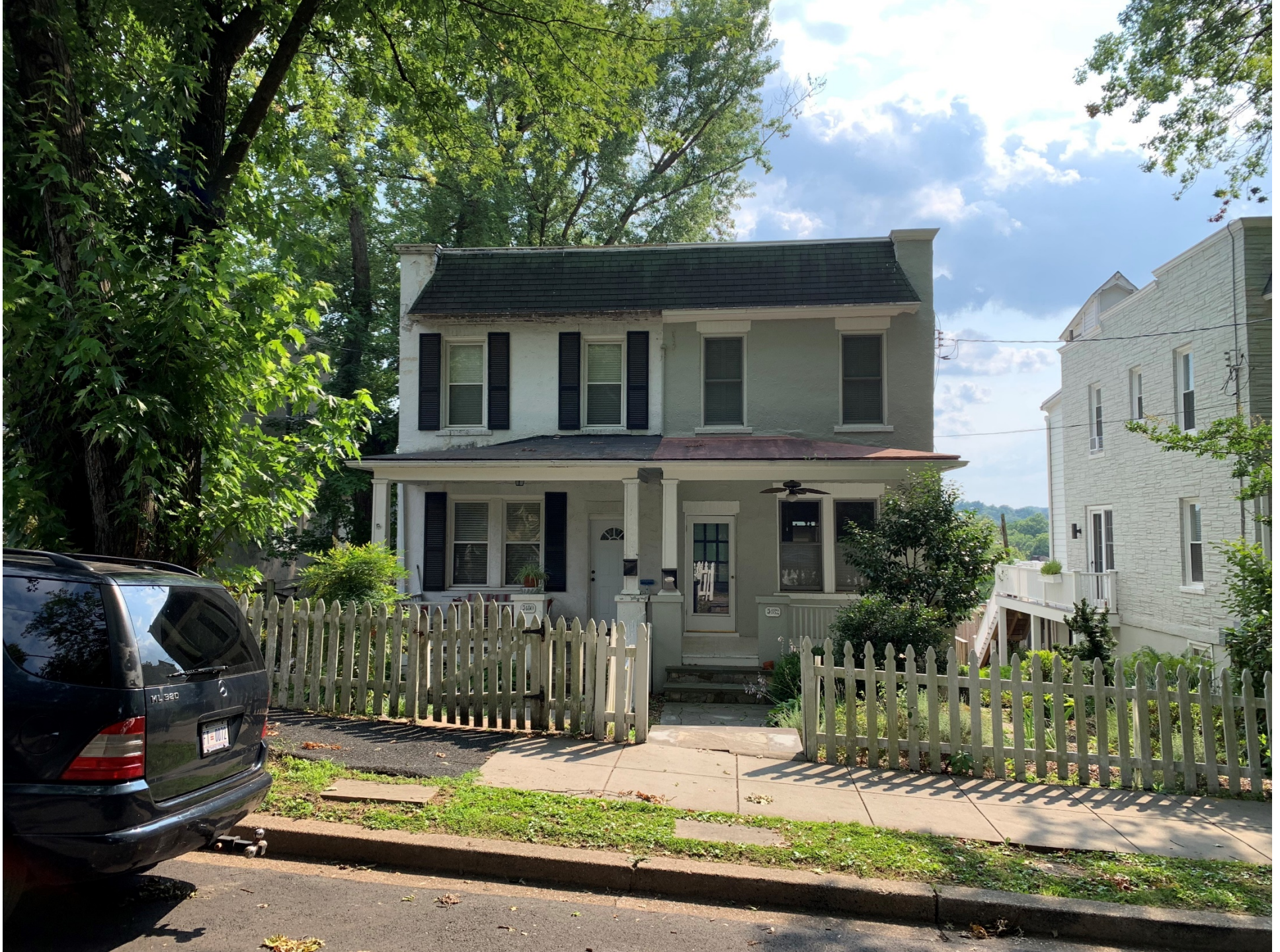
5182 Fulton Street NW House on the right
